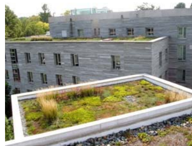
A green roof will absorb rainwater for slow release
