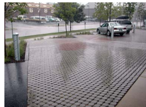
Pervious concrete block during a storm
