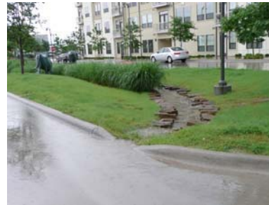
Stormwater is channeled into a sculpted watercourse instead of conventional pipes
